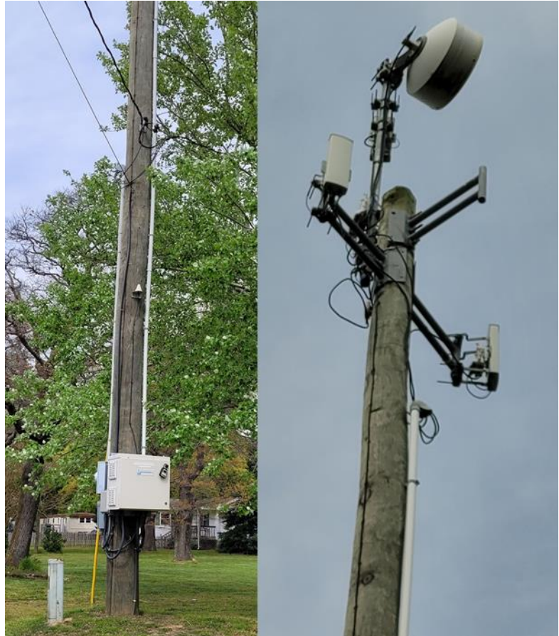
Figure 11 Neubeam Microwave Antenna, Local Antennas and Service Box Serving Smith Beach
