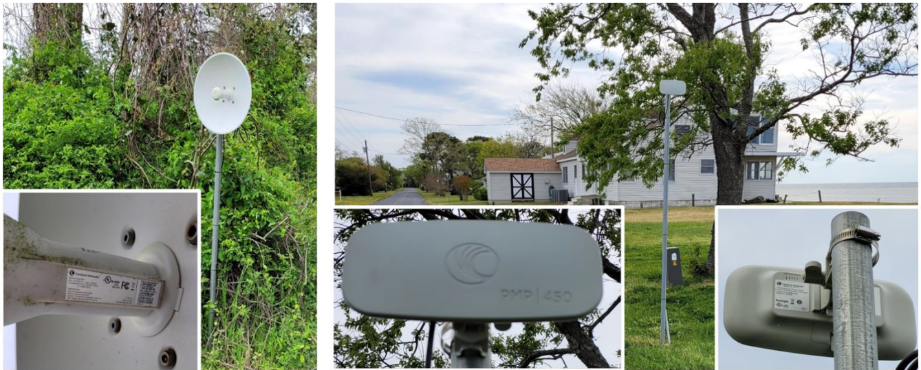
Figure 12 Typical RF to Home (RFTH) Residential Installation – a 6' Pole with a Directional or Flat Panel Antenna
