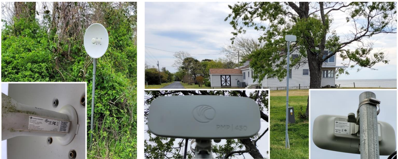
Figure 11 Typical RF to Home (RFTH) Residential Installation – a 6' Pole with a Directional or Flat Panel Antenna
